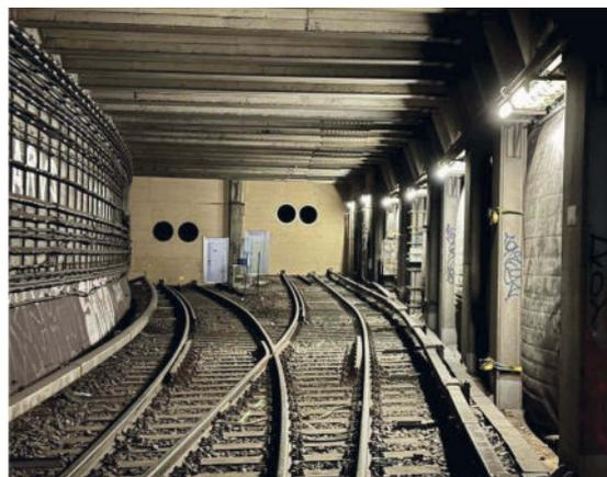
**Fig. 5:** Air separators seal off the dusty working zones from the rest of the tunnel.
