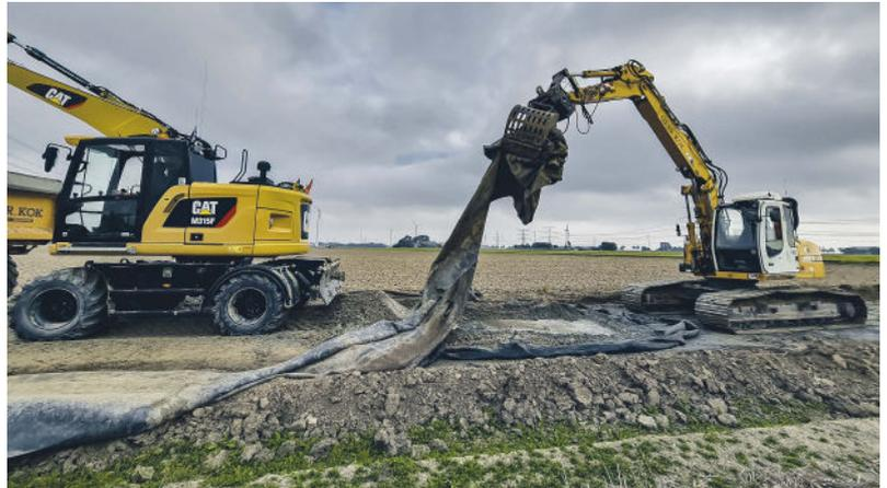
**Fig. 1:** Disassembling the temporary access road constructed for the SWITCH project
