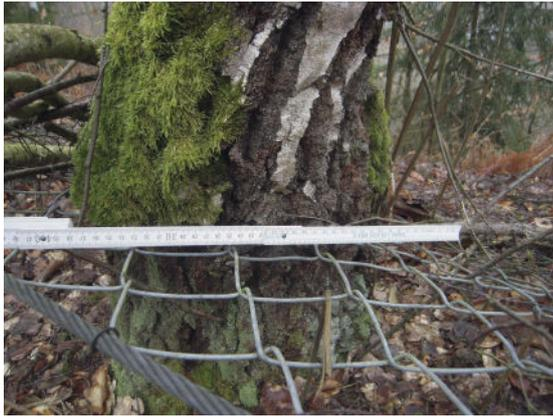
**Fig. 3:** Netting fully integrated into the tree trunk
