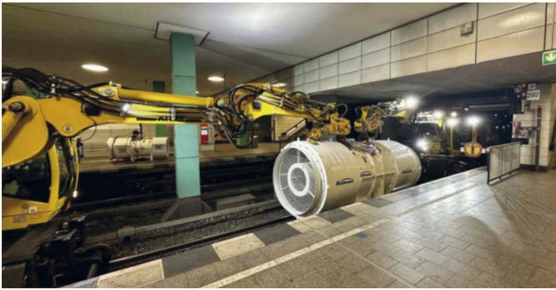
**Fig. 2:** Two-way excavator positioning a fan unit during the preparation phase.
