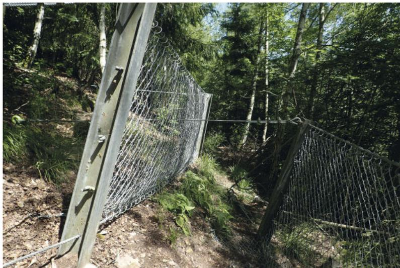
**Fig. 2:** Refurbishment of the structure – supports from the 1980s with new netting
