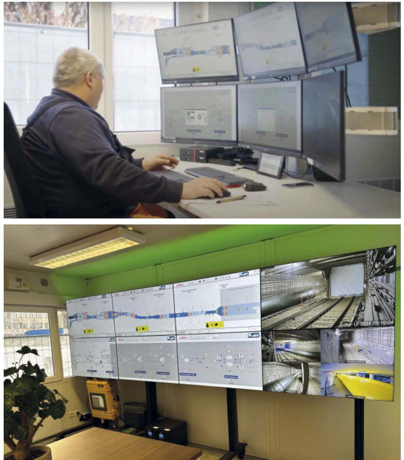
**Fig. 7:** The central control room with its data display screens is able to send commands to the on-site fans and monitor the personal tracking system.
