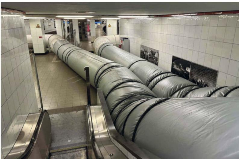
**Fig. 3:** Section of ducting for the active venting of waste air via a discharge stack at Potsdamer Platz station
