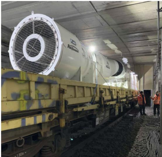
**Fig. 6:** CFT dry dedusters with a Korfmann axial fan for cleaning dust-laden waste air from the worksite
